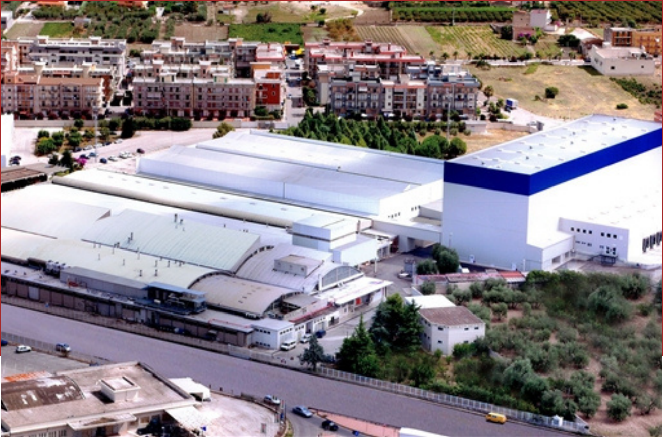
Granoro pasta factory plant in Corato (Bari, Italy)
